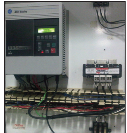
Variable frequency drives are increasingly used as a way to lower energy costs, and as a way to increase the precision of a process control system.
