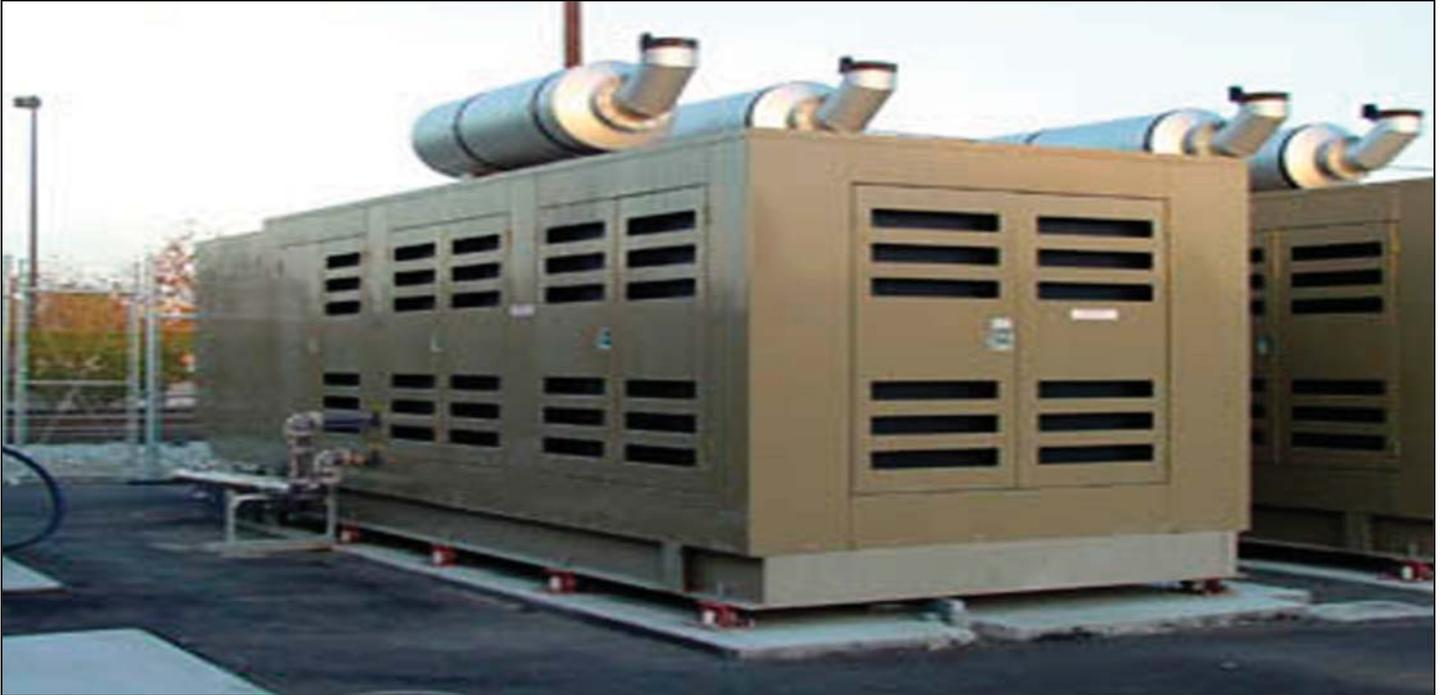
**Motor-Generators Set** – Consists of an electric motor driving a generator with coupling through a mechanical shaft. This solution provides complete decoupling from incoming disturbances such as voltage transients, surges and sags. Motor-Generators ride through short periods of power loss, but will not protect against sustained outages without the addition of an additional motor powered by an alternate fuel source (such as diesel or propane).
