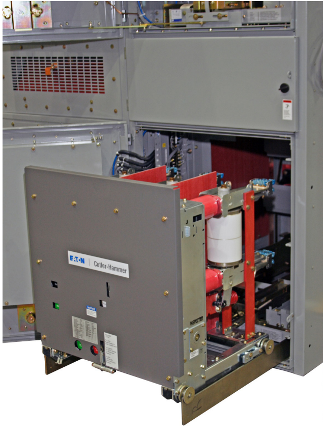
Figure 2. Medium voltage breaker racking.
